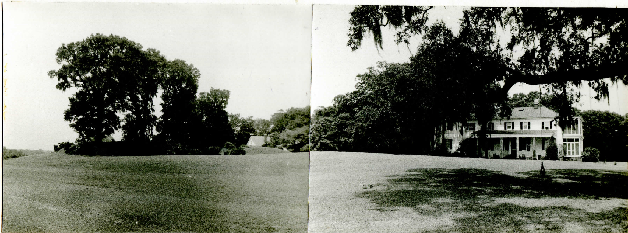
Figure 3. Photograph of the Lane yard showing the house and a portion of the Civil War fortifications.
