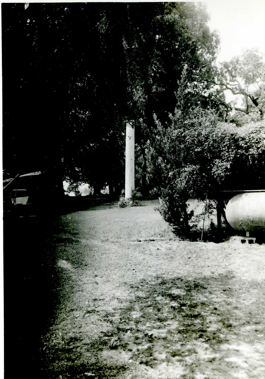
Figure 5. Photograph of the remaining column of the Christ Church, Wilton Bluff, dedicated in 1836.
